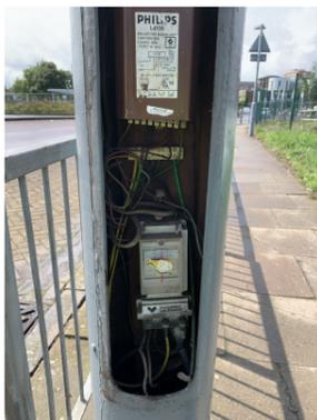
Existing Lighting column 35 has no room within the cut-out or column for extra cable to feed ANPR feeder pillar.
