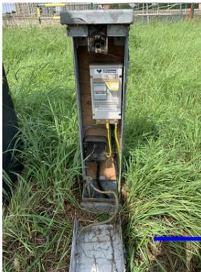
Other option for Supply is from the mini feeder pillar for the traffic lights this is only 6m away from ANPR location. if we cant run private cable from the distribution board in this feeder pillar then other option is to ask DNO to run other cable from their cut-out to new feeder pillar.
