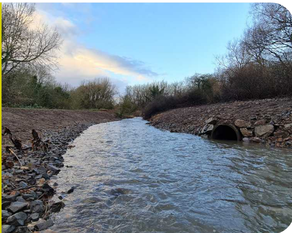
Figure 17: River Rea following channel reprofiling and removal of an engineered weir
