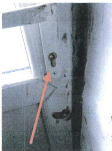
Picture 11 Replace standard lock on door Exit from kitchen with thumb turn lock to allow exit without the use of a key
