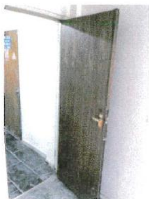
Picture 10 Replace standard door with FD 30 (kitchen)
