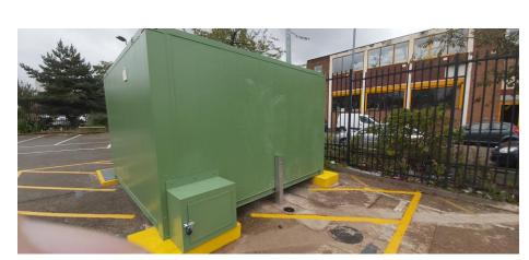
To the rear of the cabinet is a stand pipe for water (insulated silver box) which is closed and locked until pitches are rented and then the box is opened and a tap is fitted. The other green box is the box for service meters.
