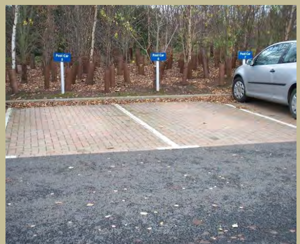
Example of permeable paving
