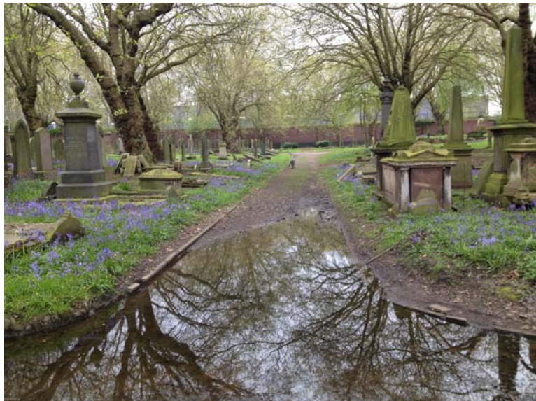
Photo of flooded path junction. The drains here require the construction of a new soakaway.
