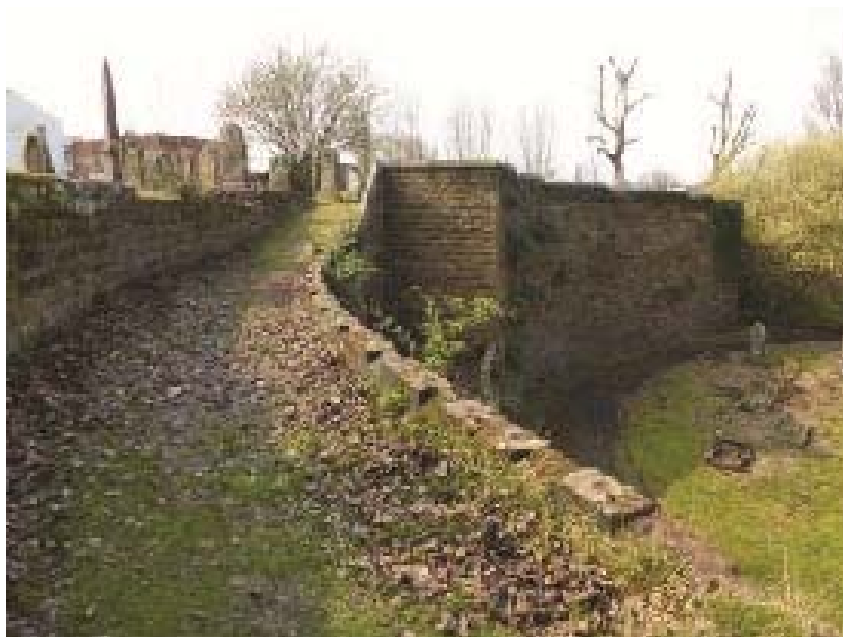
Photo from the upper level showing the poor state of repair of the wall, buddleias and the long ago removed crenulation locations.
