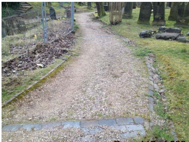
Photo of pathway leading down the side of the catacombs showing displaced gravel and silted up drainage channels.
