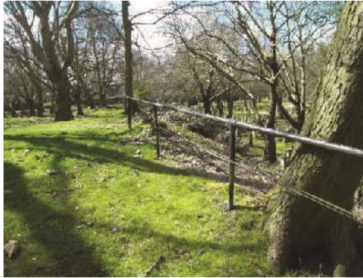
Existing unattractive scaffold bar and metal strap balustrade on the upper level
