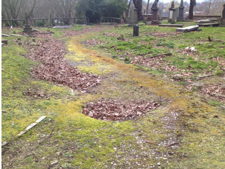
Photo of pathway above the northern Catacombs showing patches of deep potholes possibly caused by the removal of self-set trees.
