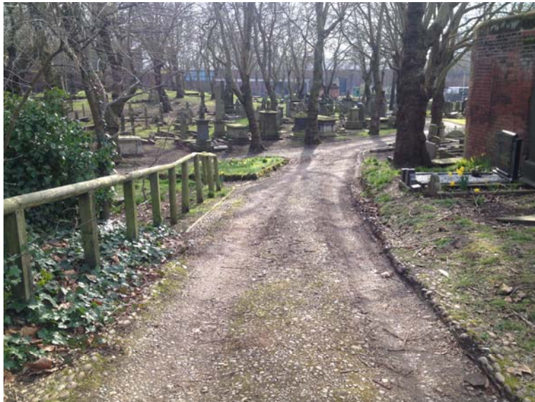
Photo of main drive leading down towards Icknield St showing ruts beside the cobble drainage strips on either side.
