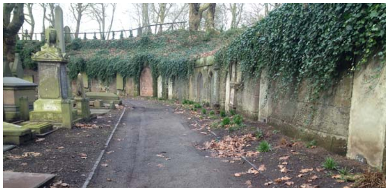
Photo showing how vegetation is undermining part of the catacomb structure. Some critical tree removals had already taken place when this photo was taken.
