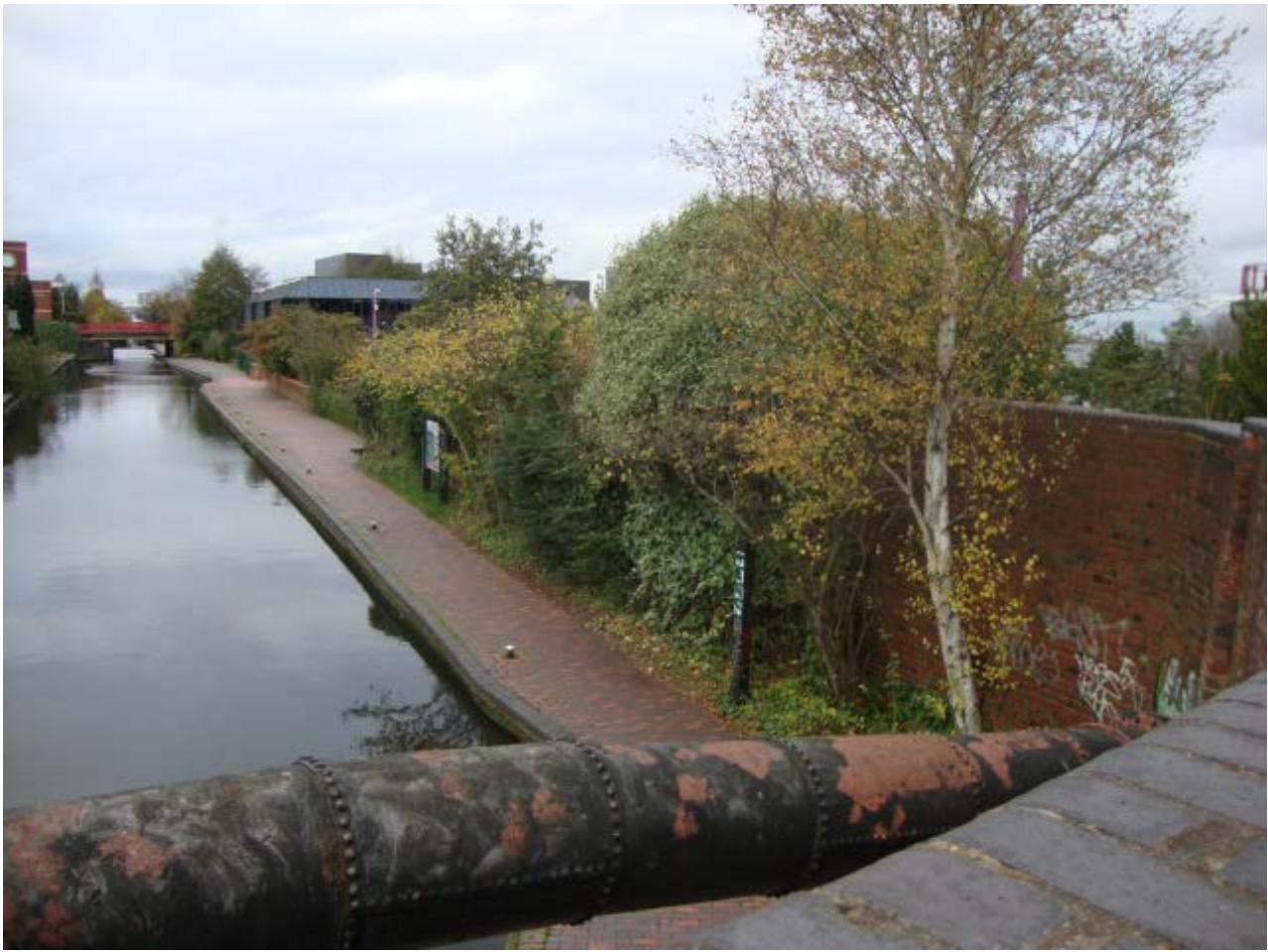
View from pedestrian bridge looking north
