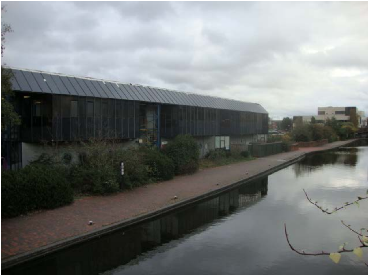
View from bridge over Canal at Lister Street
