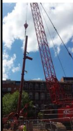
Lifting the drop-pipe and setting it in the shaft
