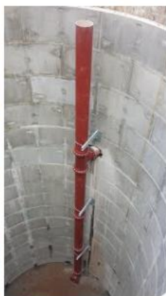
Lifting the drop-pipe and setting it in the shaft
