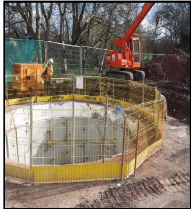
Ripple Road surface water pumping station under construction
