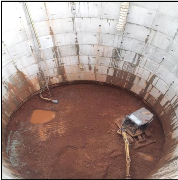
Pershore Road foul water storage tank under construction 14m diameter. 400 cubic meter storage capacity
