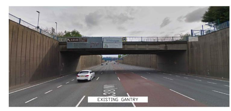
EXISTING CONNECTION TO BRIDGE FURNITURE TO BE INSPECTED BY A COMPETENT PARTY. PROPOSED SIGN INSTALLATION OF SIGN FACE TO BRIDGE STRUCTURE TO REPLACE EXISTING.
