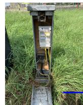
Other option for Supply is from the mini feeder pillar for the traffic lights this is only 6m away from ANPR location. if we cant run private cable from the distribution board in this feeder pillar then other option is to ask DNO to run other cable from their cut-out to new feeder pillar.
