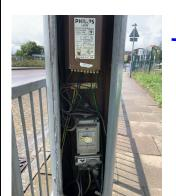
Existing Lighting column 35 has no room within the cut-out or column for extra cable to feed ANPR feeder pillar.
