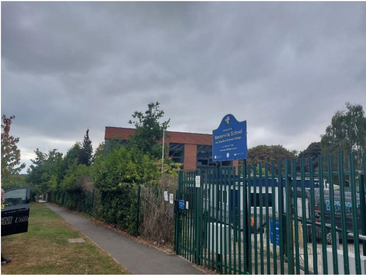
Photo 3 – Front entrance – off Fellows Lane
