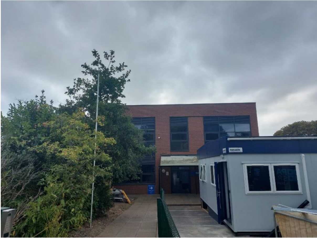
Photo 2 - Existing school building – Northern elevation at front of site
