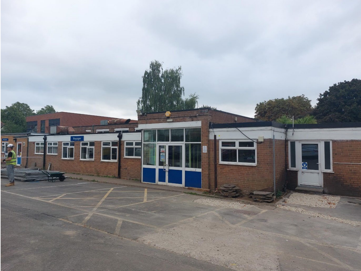
Photo 1 – Existing school building – norther elevation
