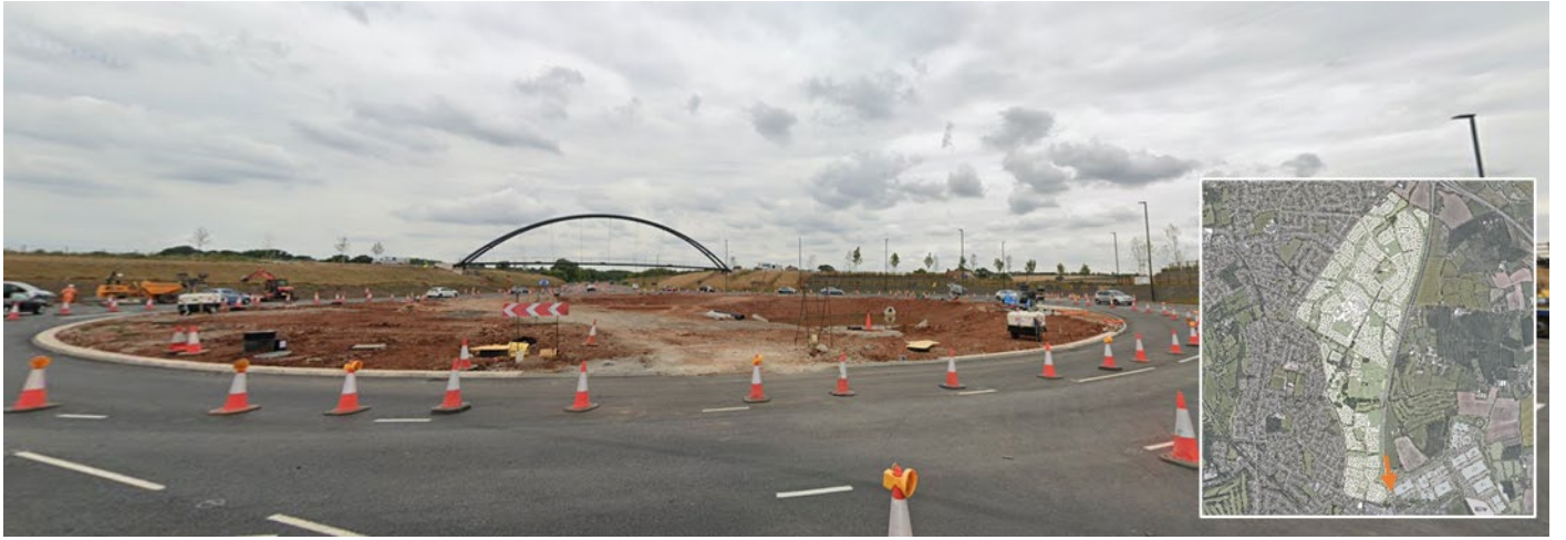
Photo 4: A38 new roundabout and pedestrian bridge (Looking Southwards)
