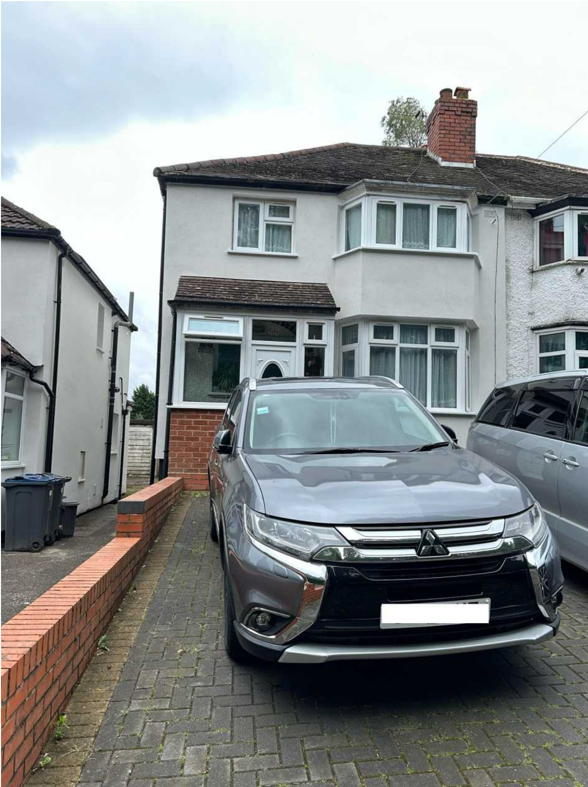
Figure 1: Front elevation of property.
