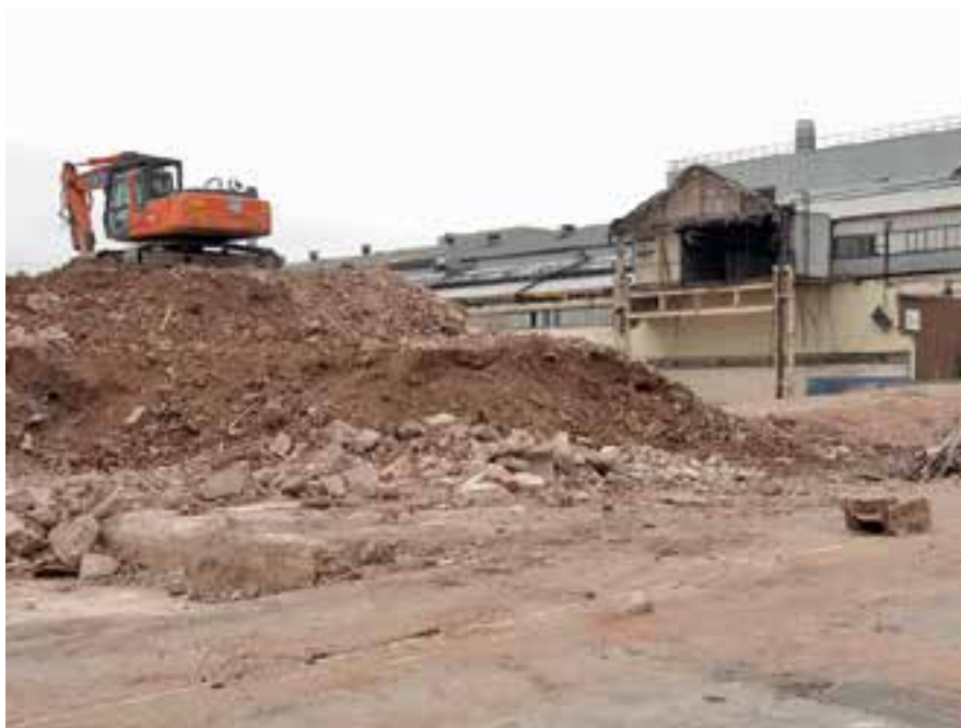
Demolition at Longbridge Page 134 of 328
