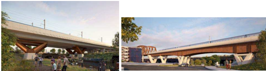
Fig 2. Comparison concrete superstructure with steel superstructure.
