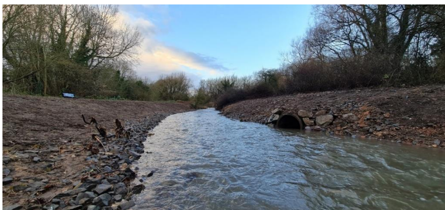
Figure 19. Re-naturalisation of the River Rea Following a Weir Removal
