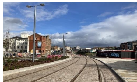
Digbeth Realm and Metro Extension
