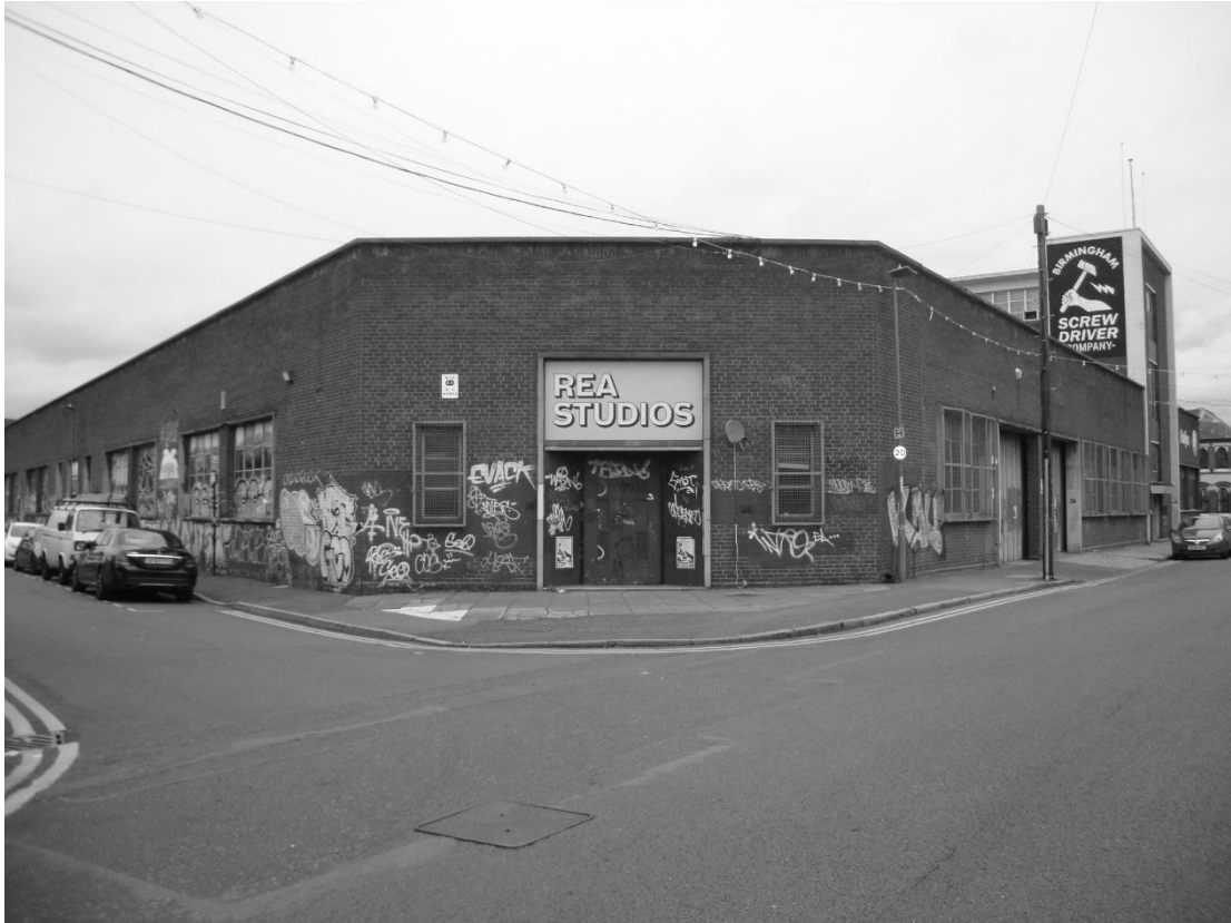
Outline Site – Rea Studios (locally Listed), Floodgate Street/Little Ann Street
