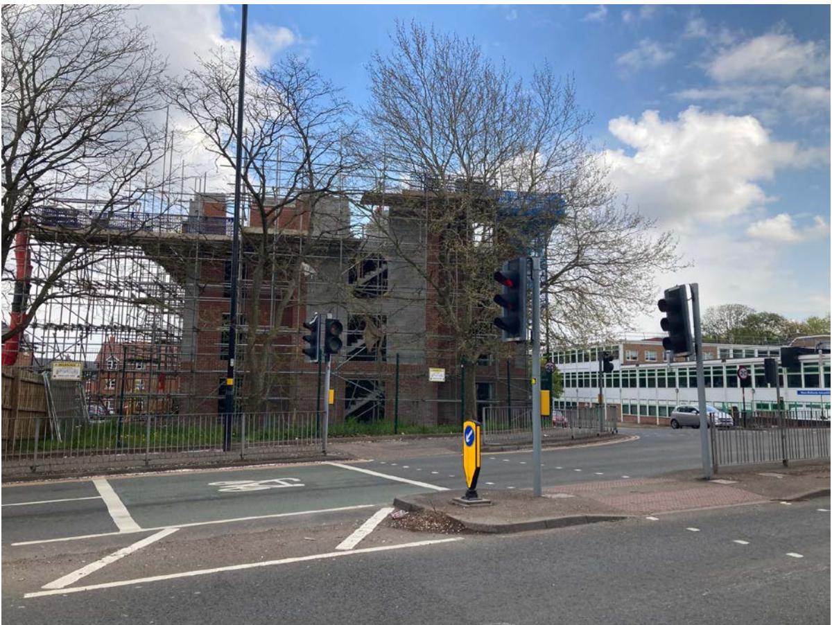
Photo 2: Oak Tree Lane elevation
