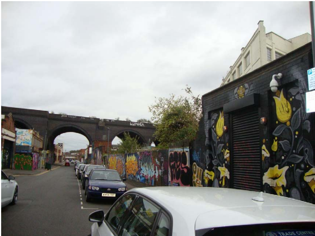
Detailed Site – Floodgate Street with Proposed Custard Factory Living (Plot CF2) to right hand side and Bordesley Viaduct in Background
