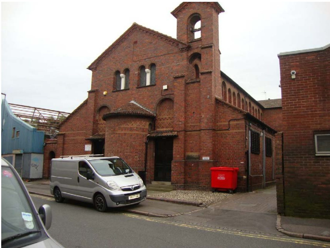
Outline Site – St. Basil's Church (Grade II Listed), Heath Mill Lane
