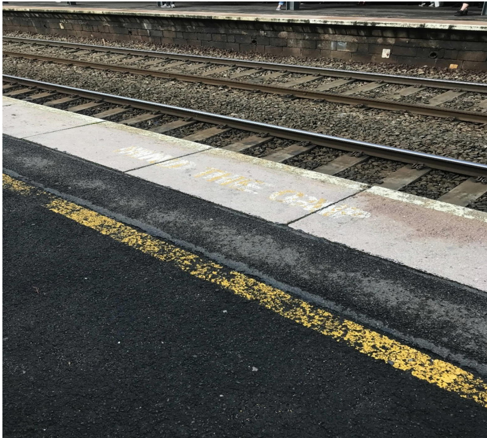
Figure 4: University Station platform with no tactile paving
