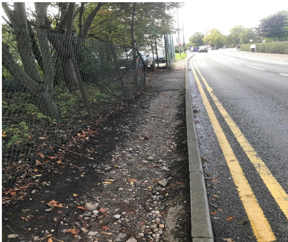
Figure 3: Poor pavement condition outside University Station
