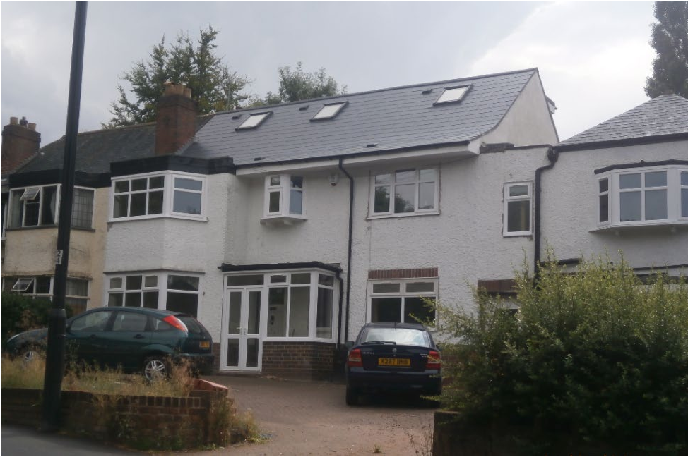
Gabel to Hip roof alteration and reduction of rear dormer in a conservation area:
